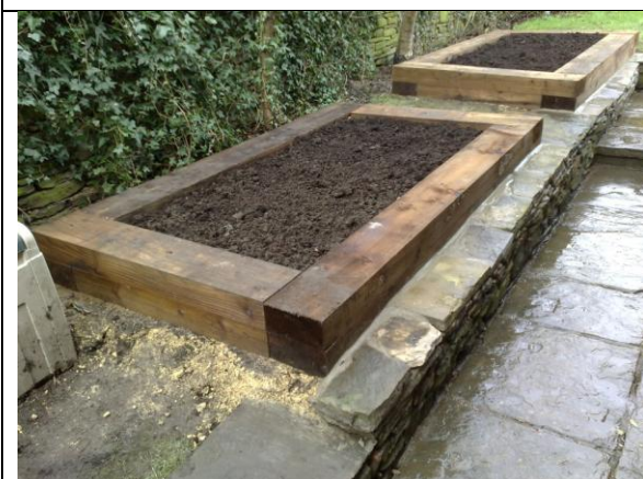
Completed planting beds using new Sleepers
