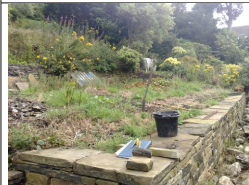
Area for raised patio using Indian Sandstone flags
